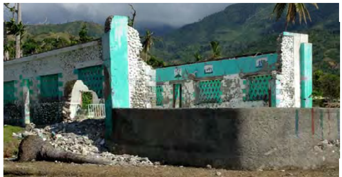
Photo: St. Josephs Church days after Hurricane Matthew. The church was considered to be a complete structural loss.
