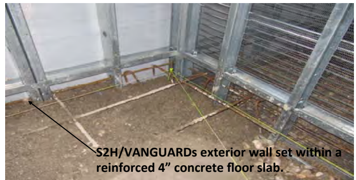
Photo: Wall Panels set within the structural concrete floor slab.
