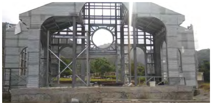
Photo Below: The exterior of the Narthex is prepared for the Exterior Structural Stucco Finishes.
